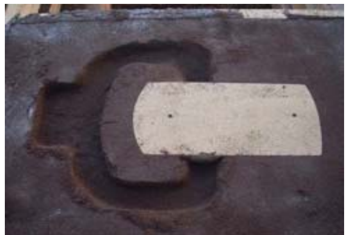
With Gate Removed Photo by R. G. Sparber
